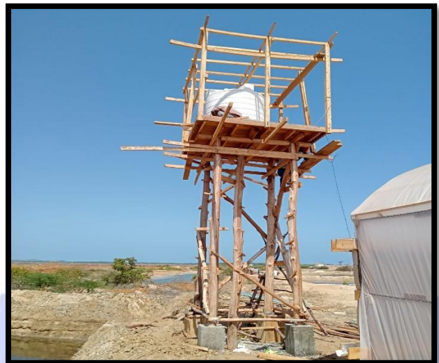
Seawater greenhouse under construction in Kilifi
