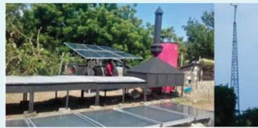
5. Hybrid windmill solar tunnel dryer: 24-hour drying fish/ farm produce; Integrated ice production unit
